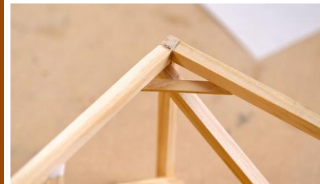
Reinforced butt joint
